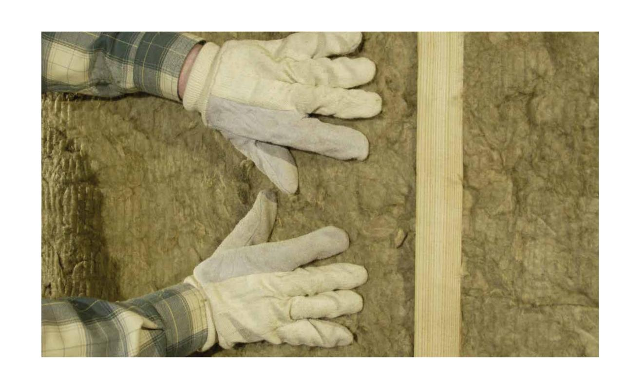
All overlaps shall be stapled at the other side of the blanket by applying adhesive tape of at least 50 mm wide.
